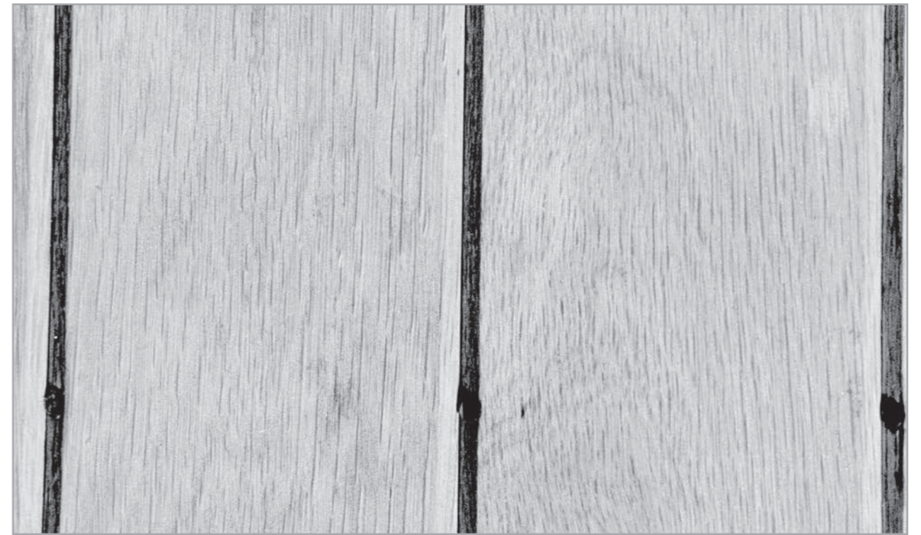
Close up of cladding - note stainless steel ring-shank nail fixing in v-joint; one fixing per board per batten.
