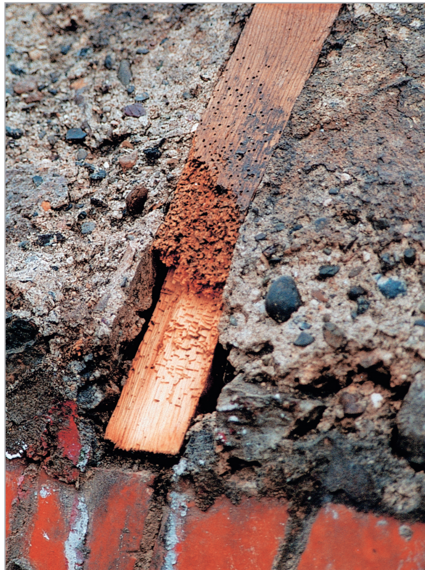
Woodworm infestation of roof rafter at eaves. High moisture content due to restricted ventilation.
