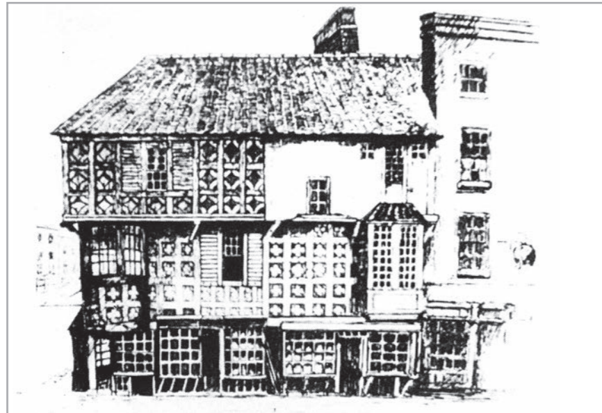
Fig. A 15.1 An historic illustration of the last recorded urban timber-framed historic building in Ireland. Note the angle posts and jettying of the upper floor, the various expressions of bracing, and decorative quatrefoil panelling on the second and third floors similar to extant buildings in Lancashire, Essex, and Shropshire in Britain. This illustration shows a shop and house built by Nicholas Bathe on the corner of Shop St. and Laurence St. in Drogheda, Co. Louth. It was demolished in 1824.
