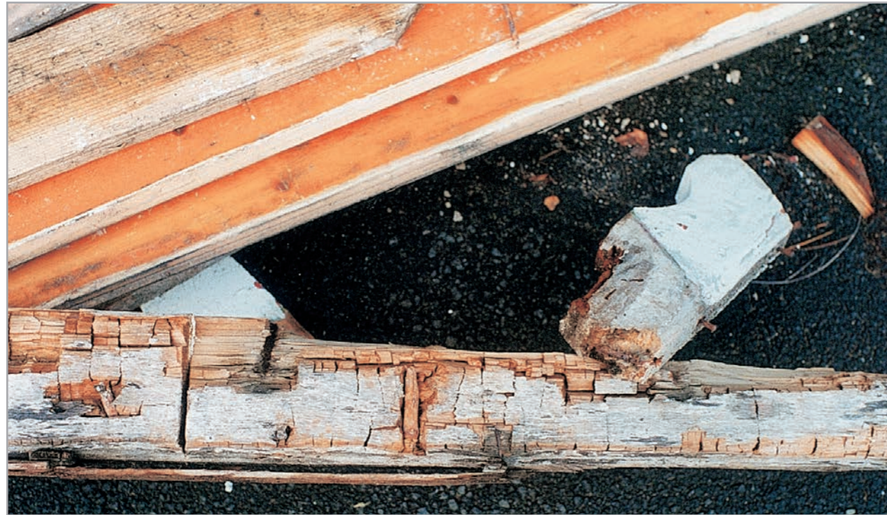
Dry rot damage to roof rafter caused by water and lack of ventilation.
