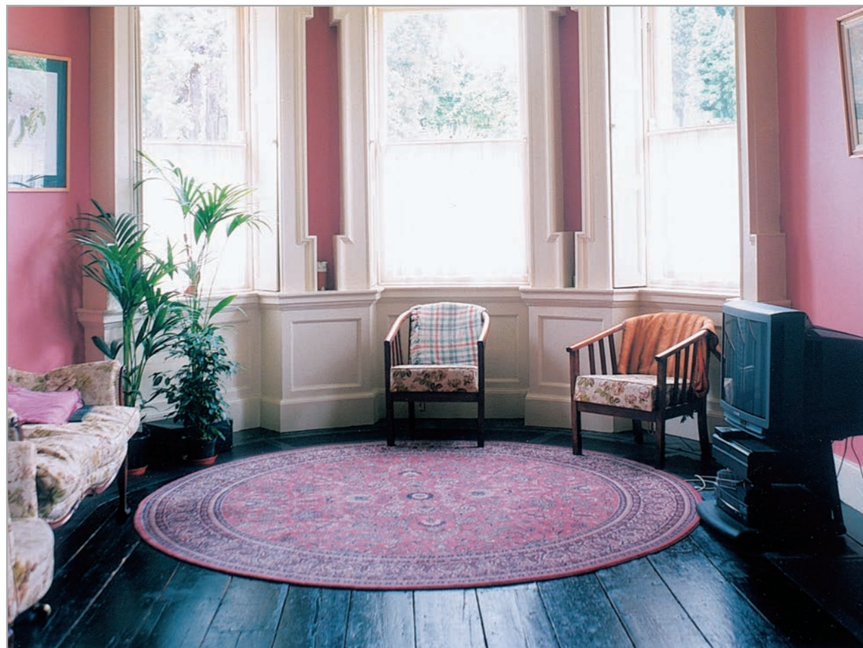
Wide square edged floorboards with a black painted finish are common in many 18th and 19th century heritage and buildings.
